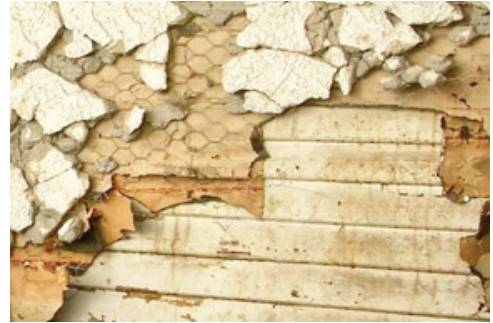
This image shows original wood siding that was incompatibly covered in stucco.
