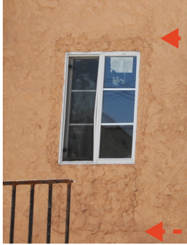
Changing window openings can leave "scars" on the exterior of a building. Red arrows indicate the original extent of the opening.
