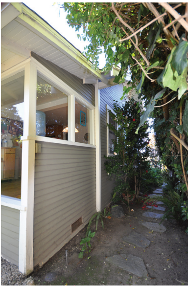
This compatible addition is differentiated from the main house by fixed single-light windows and a vertical strip of trim.
