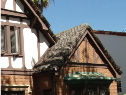
This contributor to the Bluff Park Historic District has a distinctive wood shingle roof that should be retained, repaired as needed, and replaced in kind should repair no longer be feasible.
