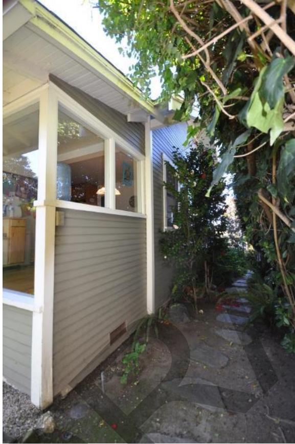
Caption: This compatible addition is differentiated from the main house by fixed single-light windows and a vertical strip of trim.
