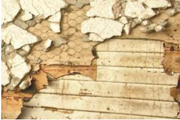
Caption: This image shows original wood siding that was incompatibly covered in stucco.
