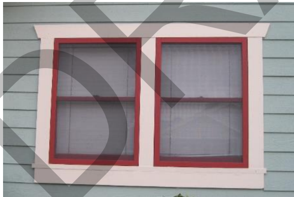
Caption: This compatible window screen is sized to the window and has a narrow wood frame painted to match the building's trim.
