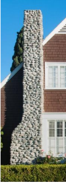
Caption: An original chimney on a contributing property in the Bluff Park Historic District.
