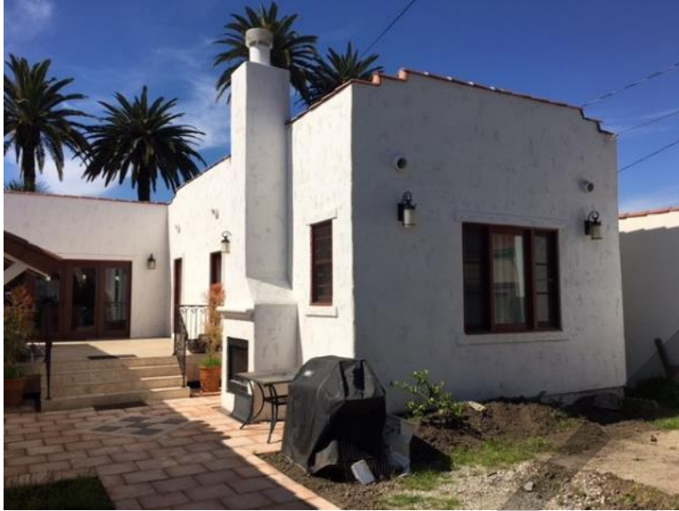
Caption: This compatible addition is differentiated from the main house with a stepped roofline, slightly different yet compatible windows, and slightly differentiated window surrounds.
